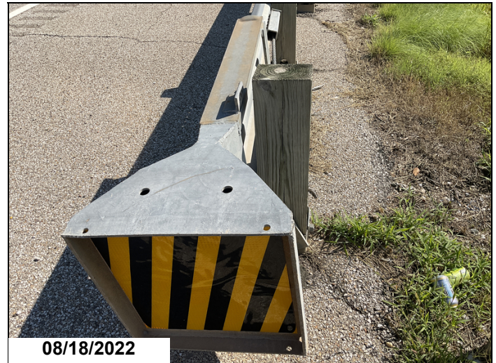
The right beginning approach railing end treatment is not attached to the post.
