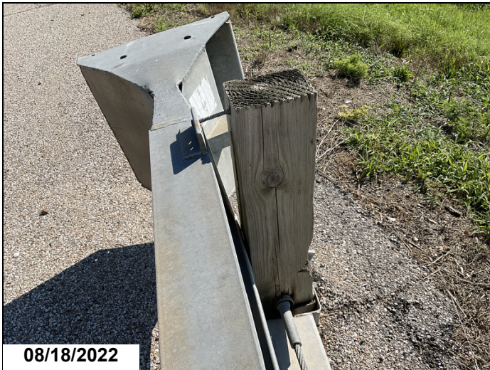
The right ending approach railing end treatment is not attached to the post.
