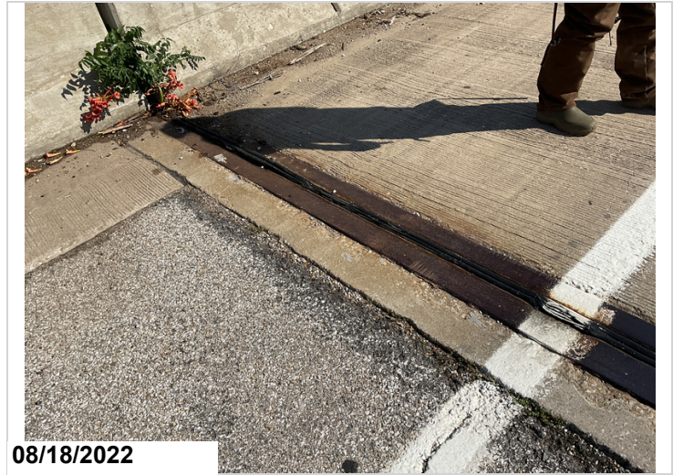
Seal damage at abutment #1.
