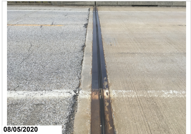
Joint seal condition at abutment 1.
