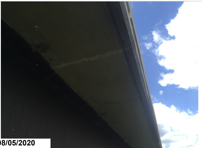
Efflorescence cracking in the deck overhangs.
