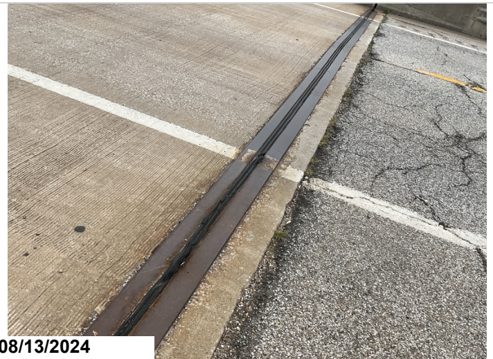
Abutment #1 seal condition.
