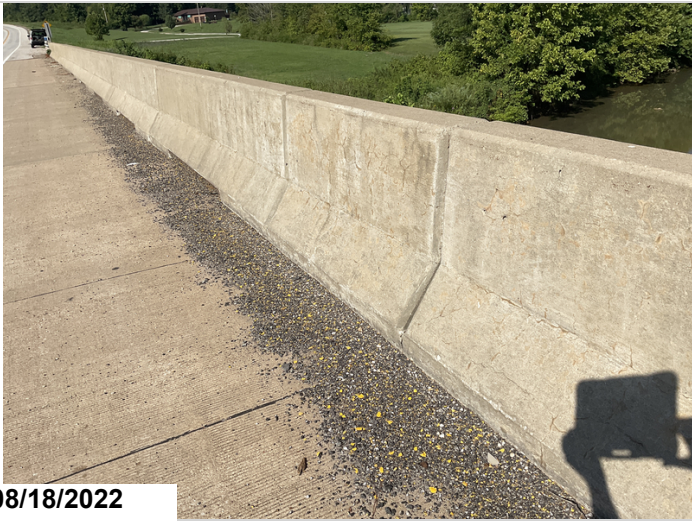
Map cracking in the left parapet wall.
